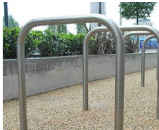
CYCLE STANDS Brushed stainless steel 'Sheffield' cycle stands to be provided in key spaces
